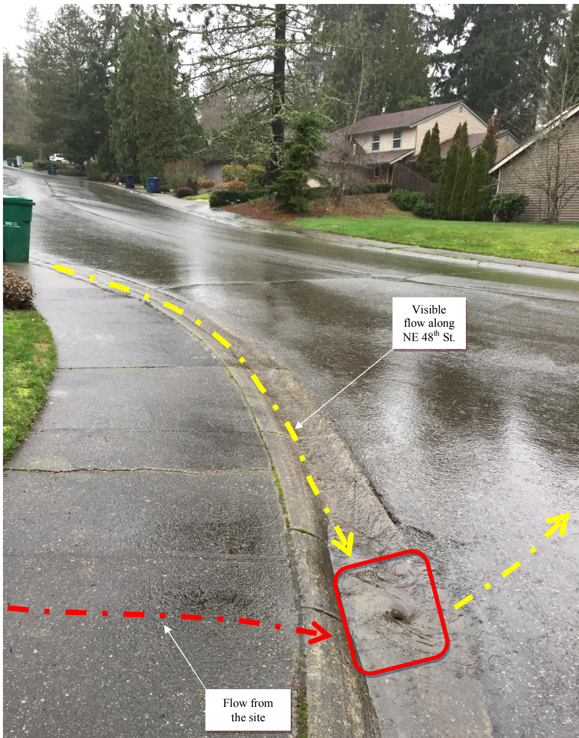
Photo 4 Current Site Condition (looking west from the intersection of the NE 48 th St & NE 48 th Ct)
